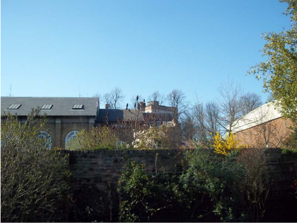
View from garden of No 112 showing the side of Founders Hall and Sport's Hall
