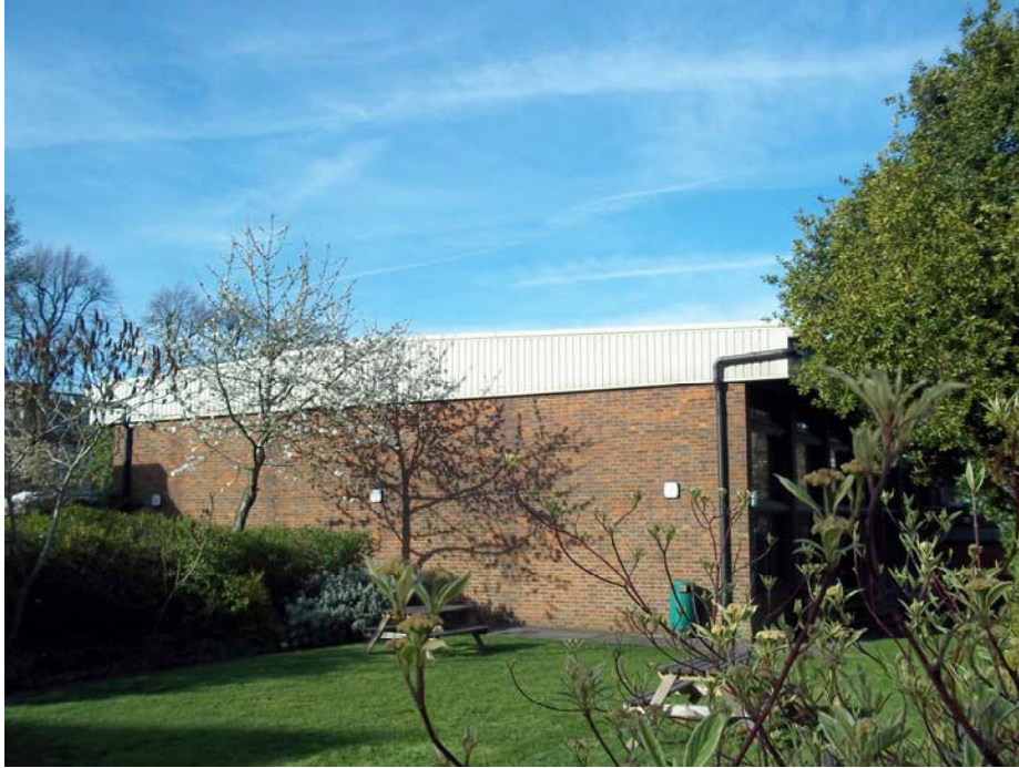
View from within the site showing front of Sports Hall
